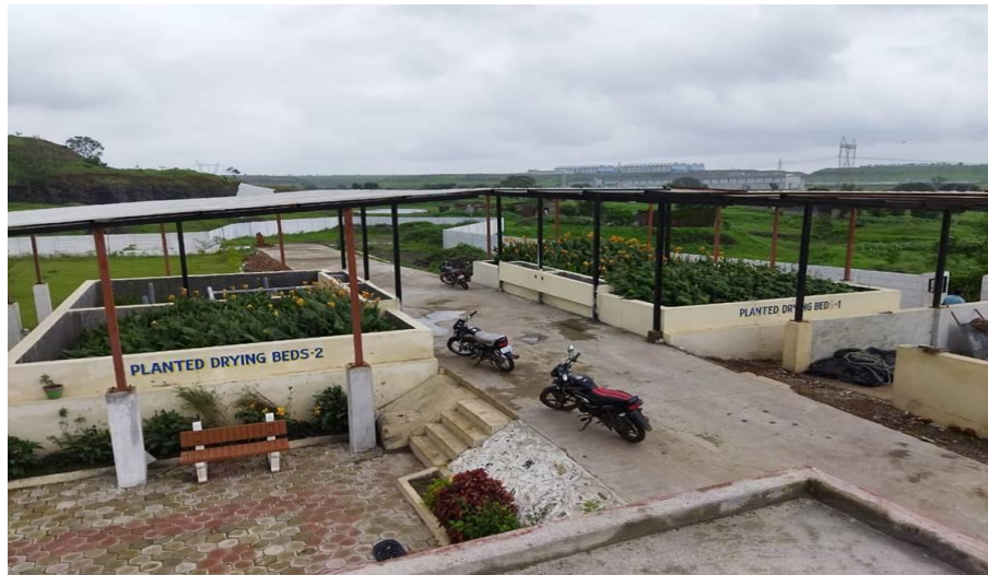
Planted Drying Bed FSTP @ Kali Bilod – near Indore, Madhya Pradesh. Courtesy – CDD India
